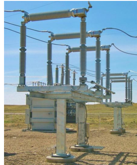
Horizontal interrupter circuit switcher
