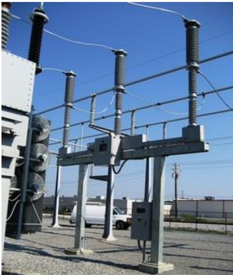
Vertical interrupter circuit switcher
